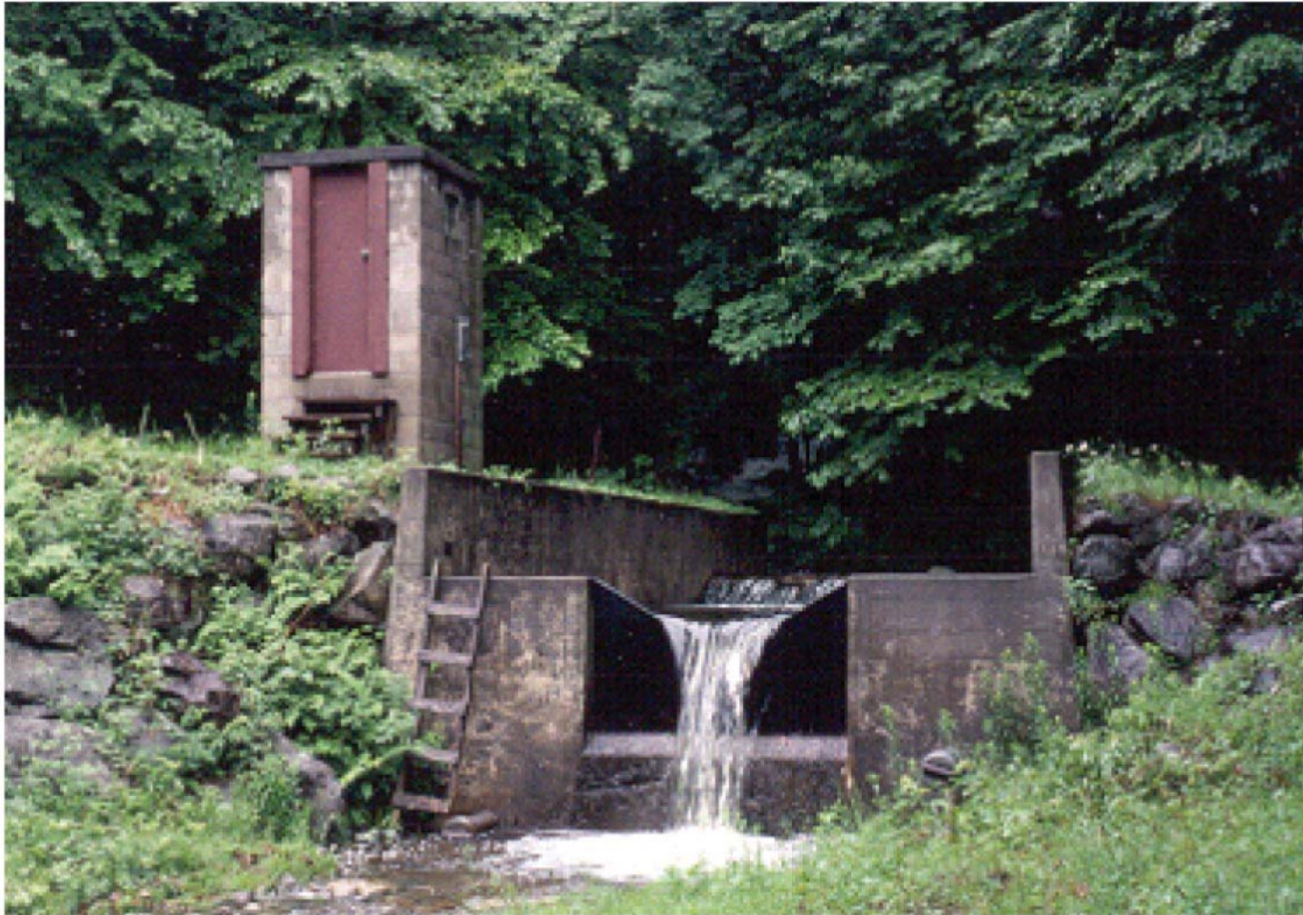
(a) Concrete dam and weir
