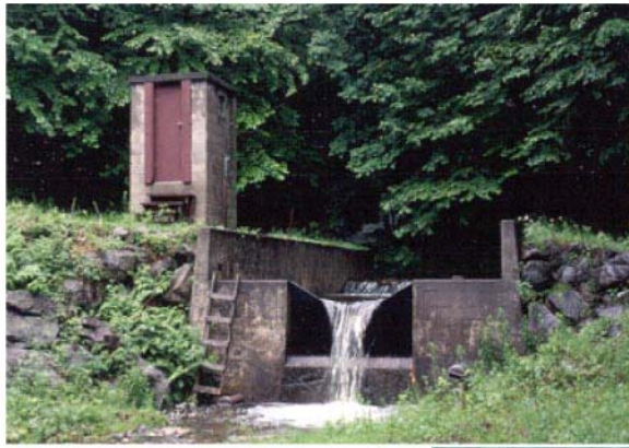
(a) Concrete dam and weir
